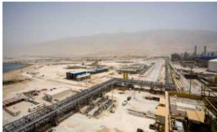
Project title: Connecting plan of Phase I and II Employer: NPC- Damavand petrochemical. Location: Assaluyeh
